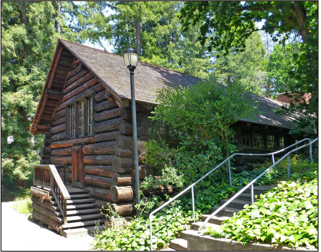
Senior Hall after restoration. Steven Finacom, 2024.
