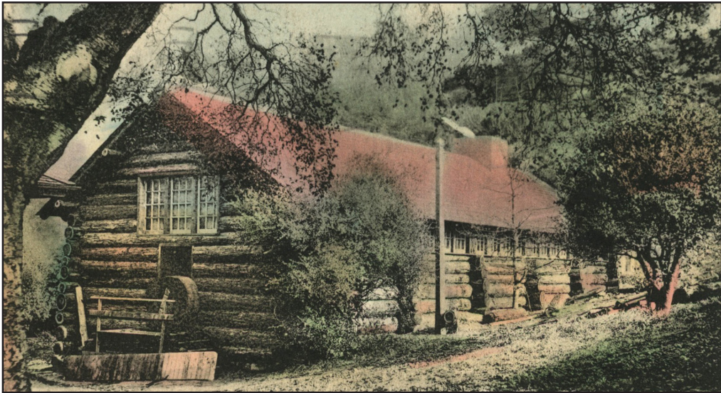
Senior Hall — construction is almost complete in this 1906 hand-colored postcard view published by local book store, N. J. Abbott & Son. Courtesy Anthony Bruce.
