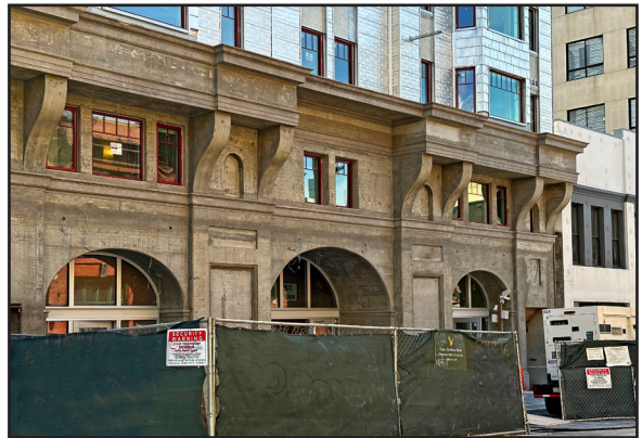
The concrete podium under construction. Anthony Bruce, 2023.
