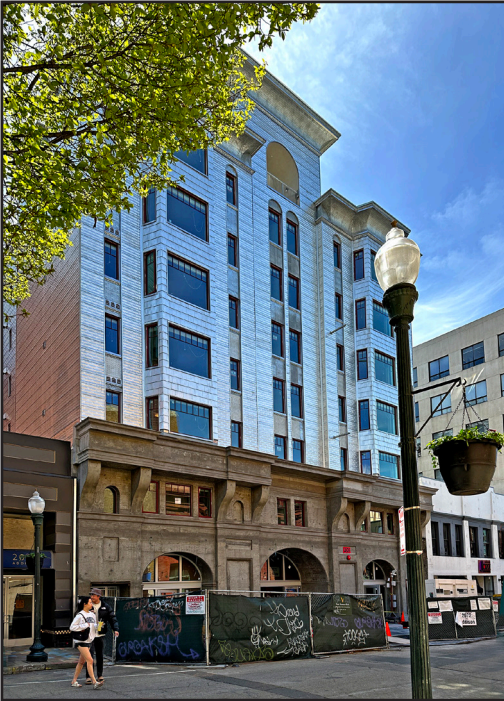
The Artisan, nearing completion. Anthony Bruce, 2024.
